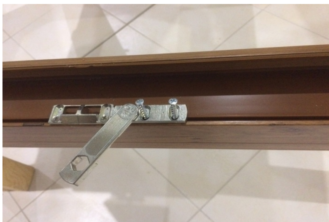
Installation des vis fournies
